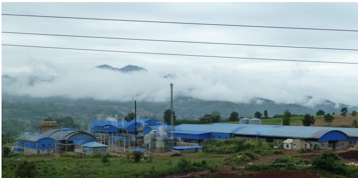
Cornerstone Zinc Refinery, Lashio, Northern Shan State, Myanmar
